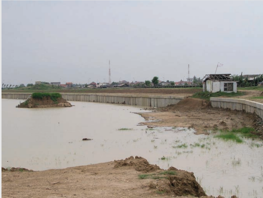
Photo 7: The island in this section of the East Canal was created as builders dug around a lot where the owner of a house had not yet received compensation. (The structure has now been dismantled.) Despite the constructors' concerns not to disturb uncompensated property, the owner could have made little use of his preserved, yet inaccessible, property.
